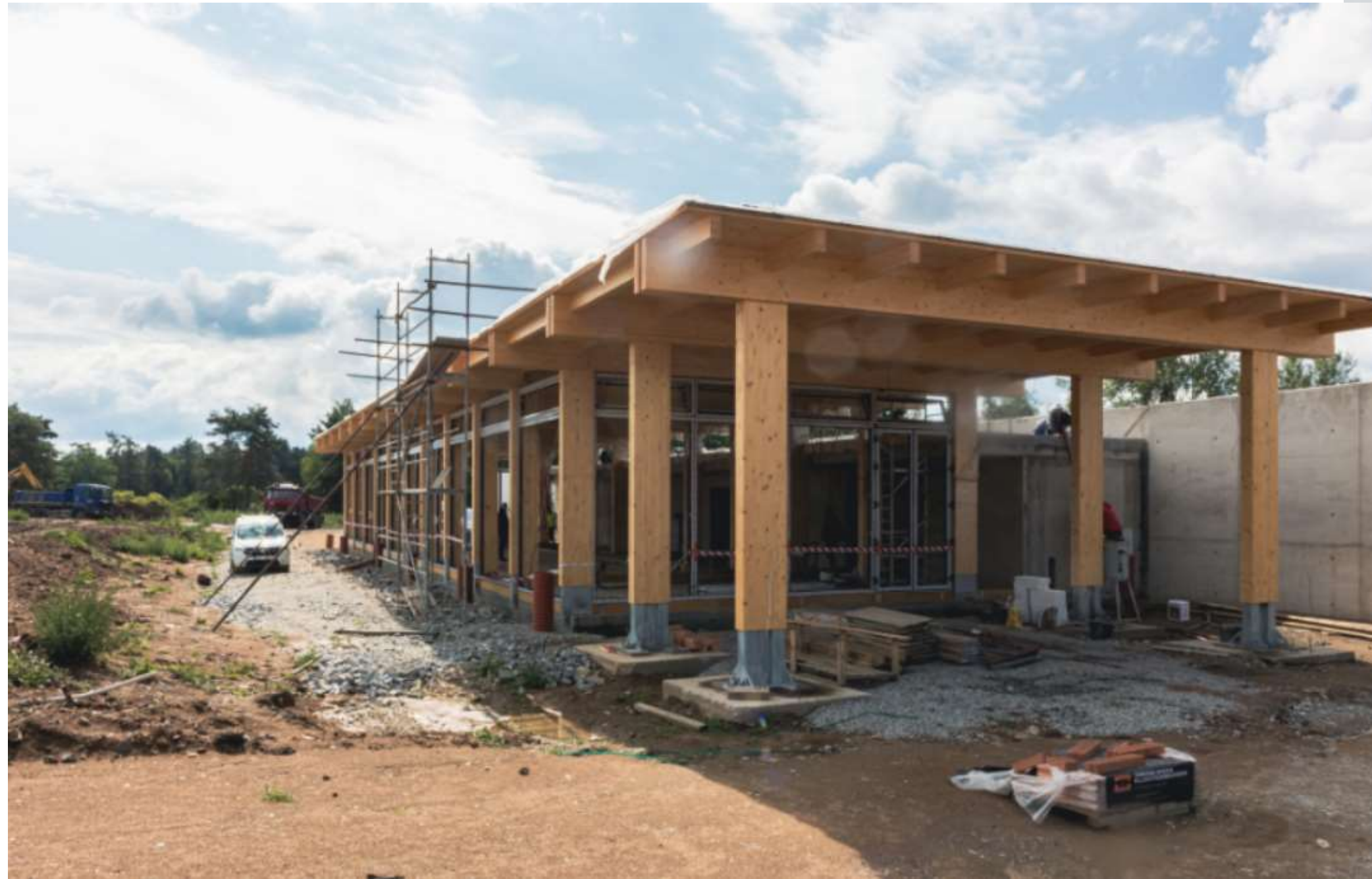
Actual status of construction works – visitors centre
